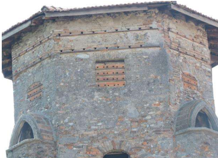
Figure 15: Two lines of cells for swifts in the upper part and windows blocked for the cells for sparrows
