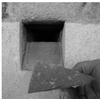
**Fig. 1** A scaffold hole modified to be inaccessible for pigeons and allow swifts and bat enter; a wedged piece of brick is shown before the use in the hole
