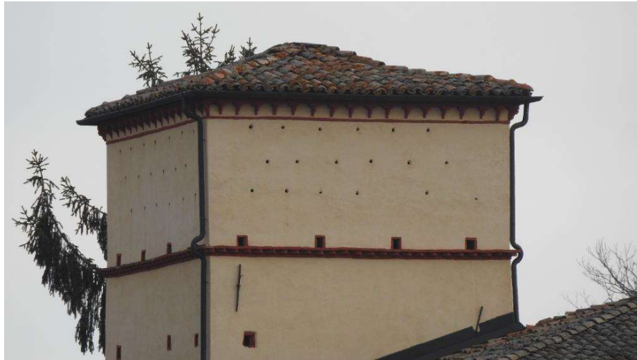
Figure 6: Tower house ( casa torre ), with little square windows for the dovecote and smaller holes for swifts, well renovated, Guiglia (MO, Italy).
