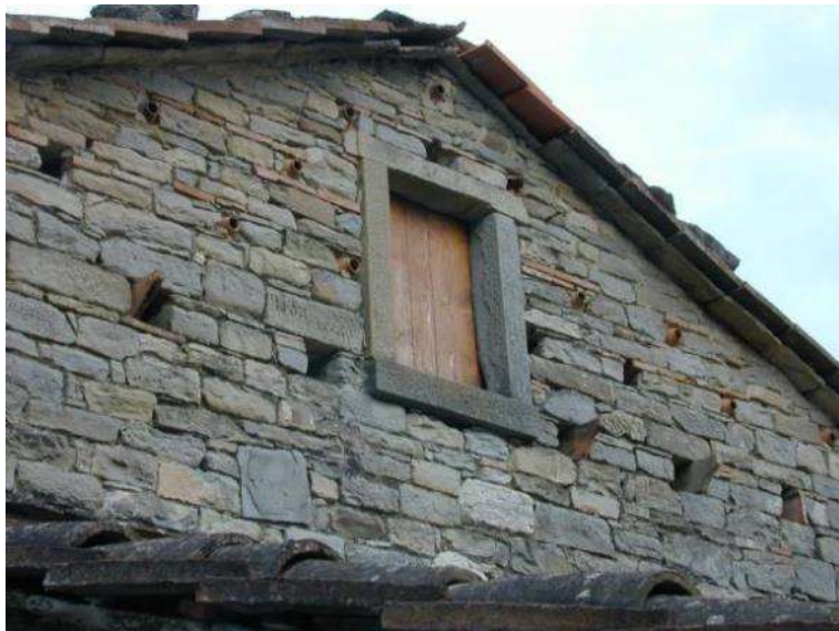
Figure 9: Swift pots partially embedded in the walls of a dwelling, Appennine of Romagna, Italy Photograph © Mauro Ferri
