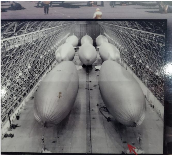
An airship at NAS Tillamook hooked up to one of the hangars' underground power stations.
