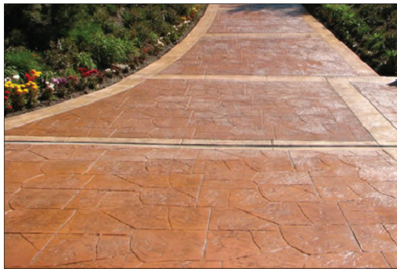
Stamped and Colored Concrete
