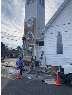
Each time we thought caulking would remedy the leak. However the leaks became more severe and we decided we needed to hire another company to take a deeper look. It turns out that the wind and rain had been able to get behind the siding causing extensive damage to the plywood panels and wet soaking insulation. It was rotted and covered with black mold.
