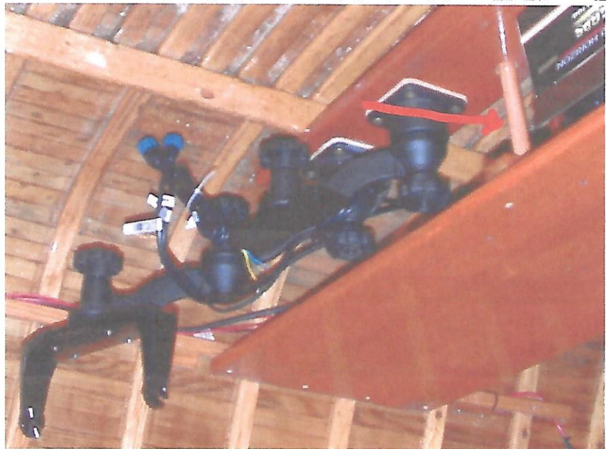
Figure 17: View of dowel reinforcement for bench seat.
