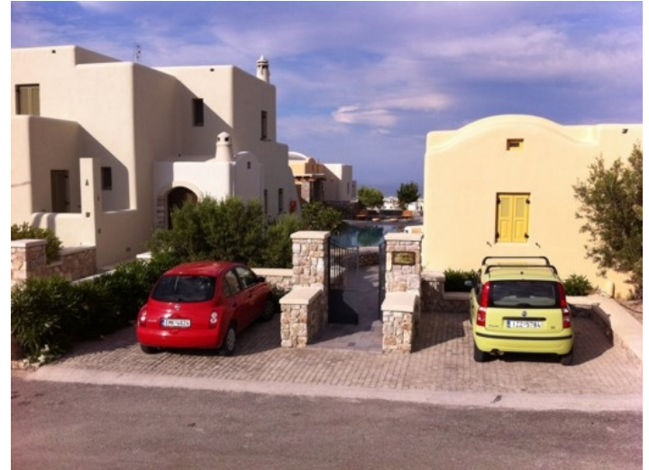
Building on left hand side, Energy classification (A-) Solar buffer tank 500 L, additional energy source oil burner
