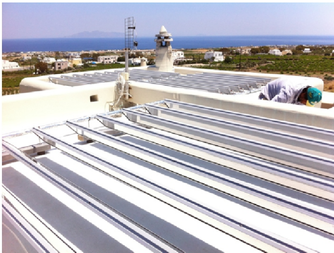
The backside of solar panels are temporarily covered by an aluminium plate which can be exchanged to PV-modules.
