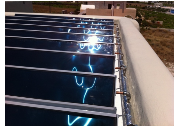
The preinsulated distributor pipe is fixed to the wall by ordinary pipe pipe fixtures with rubber surface.
