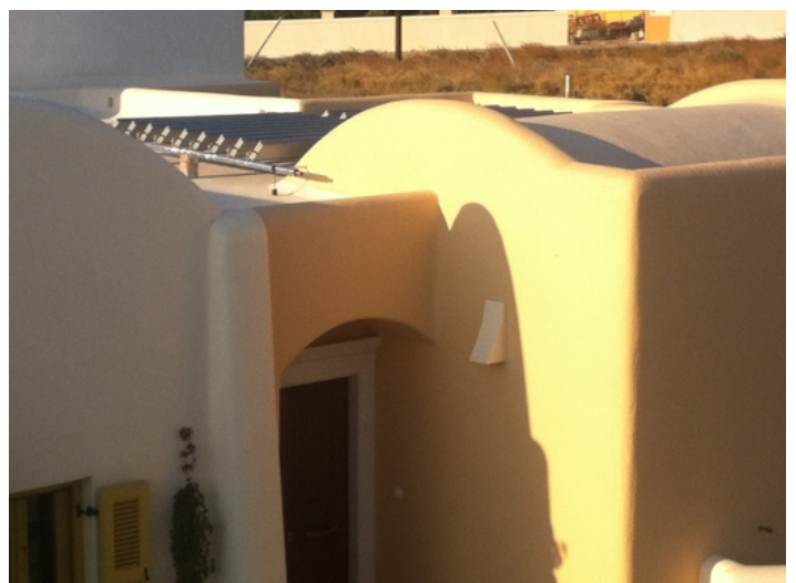
The solar panels have a very low (20 cm) 'hight profile' and are not visible from the street level.
