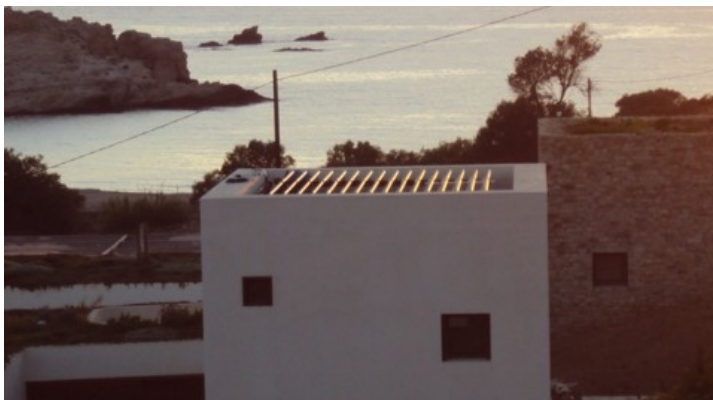
The panels does not disturb the structural arctitecture lines if symmetrically incorporated on to the roof space.
