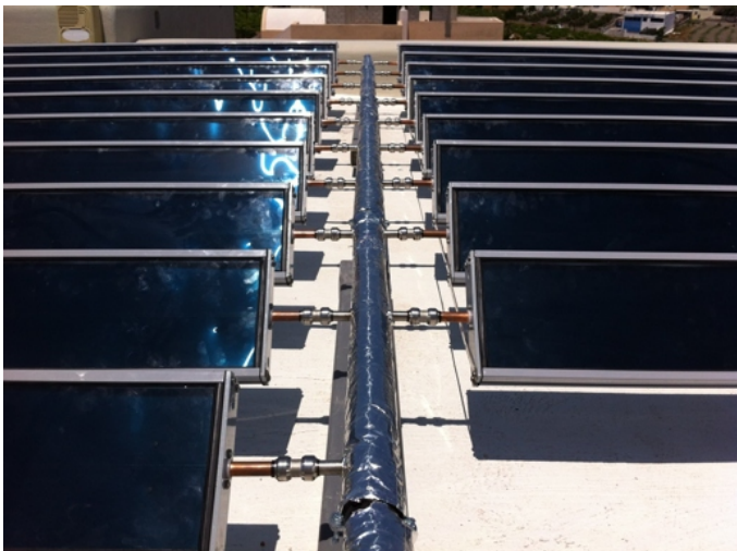
The selfbearing collecting pipes are of stainless steel 304 and the connector couplings are in stainless steel SS 316
