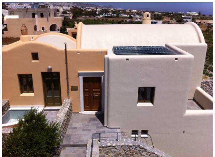
The solar panels have a very low (20 cm) 'hight profile' and are not visible from the street level.
