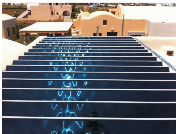
Panels can preferably be arranged in symmetric arrays. The hot water outlet pipe must higher than the inlet pipe.
