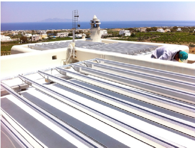
The backside of solar panels are temporarily covered by an aluminium plate which can be exchanged to PV-modules.
