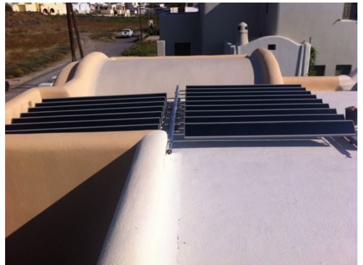
Panels can be arranged in non symmetric excentric arrays. Normally the middle double pipe is the hot water outlet.
