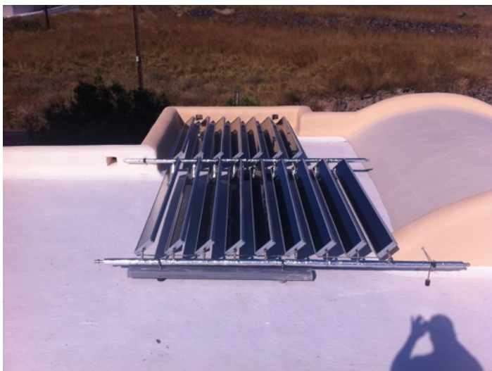
A slight inclination is necessary for open circuit systems. On closed pressurised circuits the installation can be flat.
