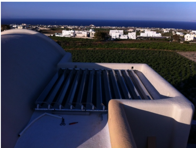
The Panels must be fixed towards a wall on at least one side, other distributor pipes can be mounted upon foundations.
