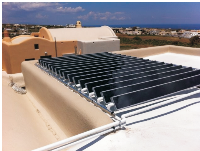
The Panels must be fixed towards a wall on at least one side, other distributor pipes can be mounted upon foundations.
