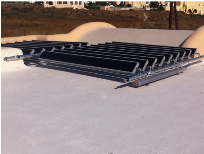
The Panels must be fixed towards a wall on at least one side, other distributor pipes can be mounted upon foundations.
