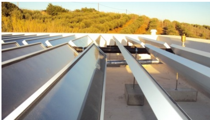
The panels are mounted on collector pipes with c/c 250 mm and are thus not affected at all by any strong winds.
