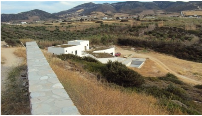
300 m2 building with Energy classification (A+)
