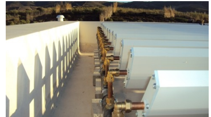
The distributor pipe can be fixed towards a wall on one side or be mounted directly on small concrete foundations.
