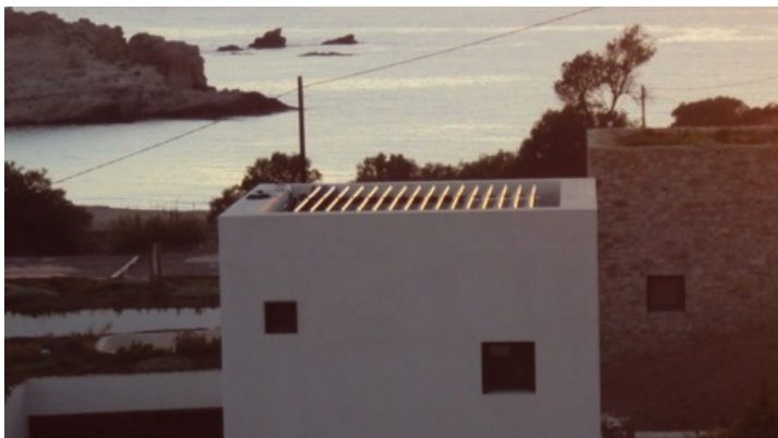
The panels does not disturb the structural arctitecture lines if symmetrically incorporated on to the roof space.
