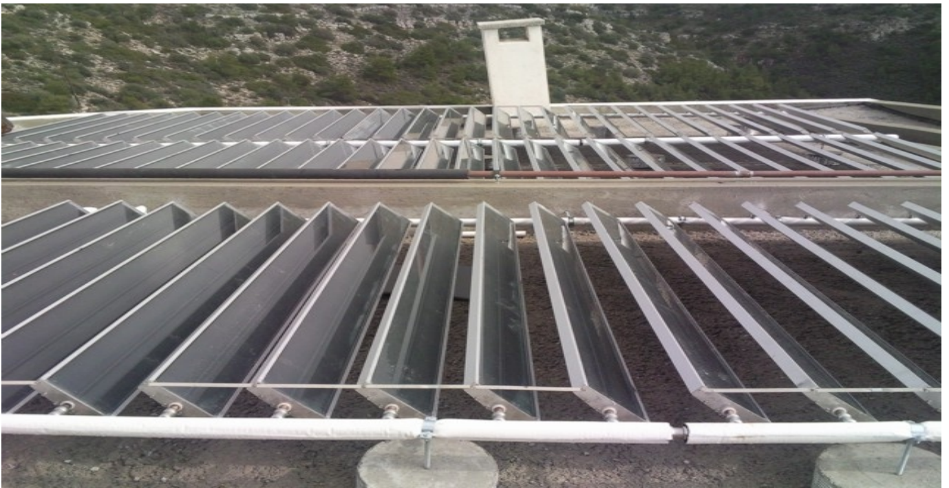
Installation on flat roof for central floor heating system, hot water and pool heating.
