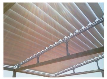
The Panels here are fixed towards special inclinable rails, with pipe fixtures holding the insulated distribution pipes..
