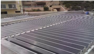
On the contrary the other supposed horizontial area (green circle) consists of multiple stripes of solar collecting surfaces with an inclination of 45' towards the horizon, effectively collecting the weak solar radiation for heating purposes during the winter period.
