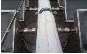
Whenever the package includes a double distribution pipe the the connections starts from the middle pipe.
