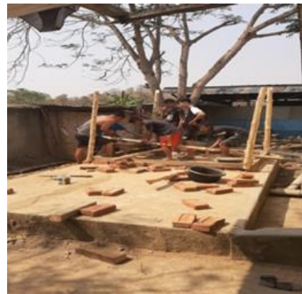
Helping with construction
