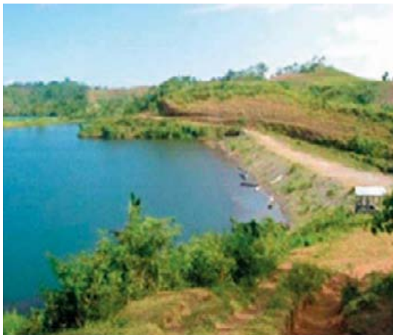
Figure 6.4. Small Water Impounding System in the Philippines
