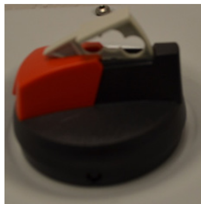
White center tab opened in OFF position with 3 padlock holes
