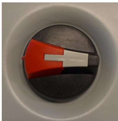
DC disconnect switch OFF position
