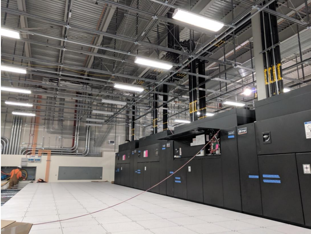
Figure: Electrical raceway, switchgear, and power systems inside T-Mobile's mission-critical facility.
