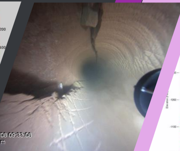
Drilled Water Intake Shaft
