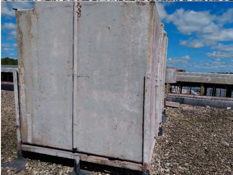
33. Gray and red on metal and fiberglass material.
