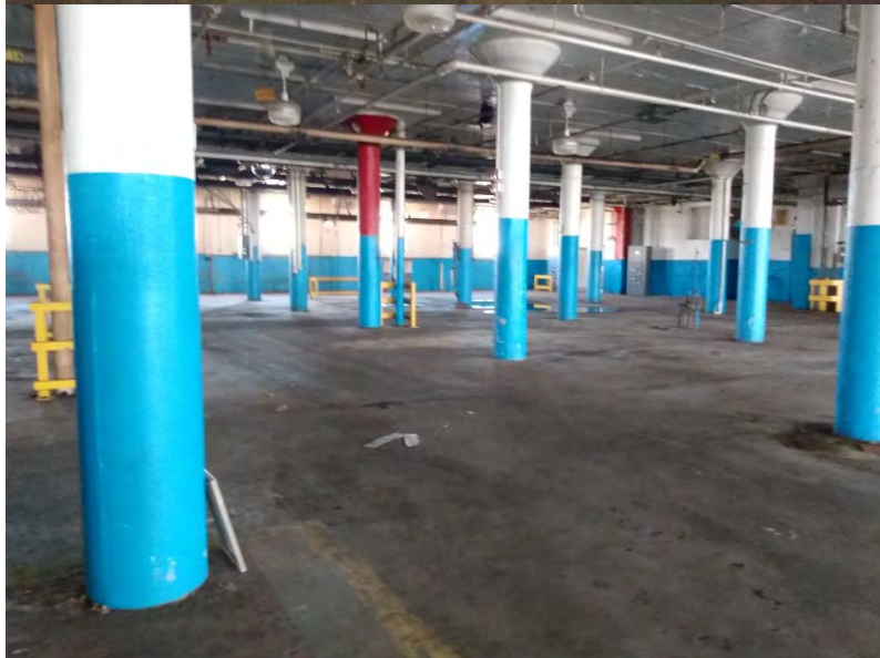
12. Blue lower half of concrete columns.
