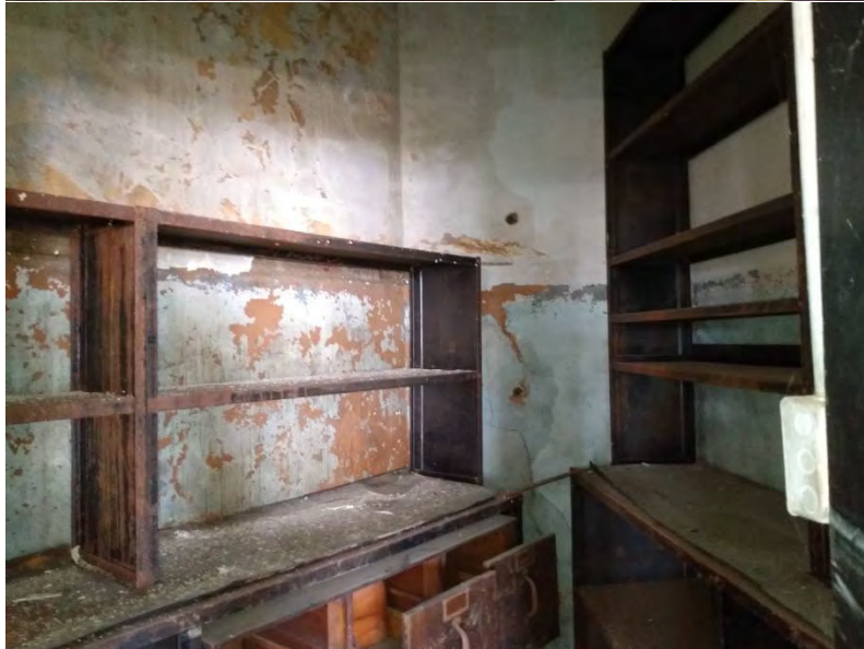
20. Blue and gray concrete wall inside the safe.
