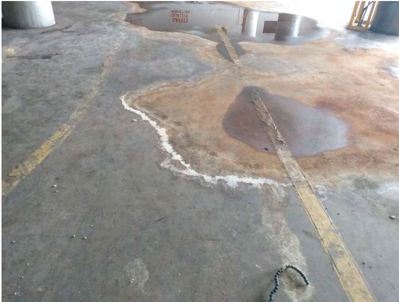
4. Yellow on concrete floors.
