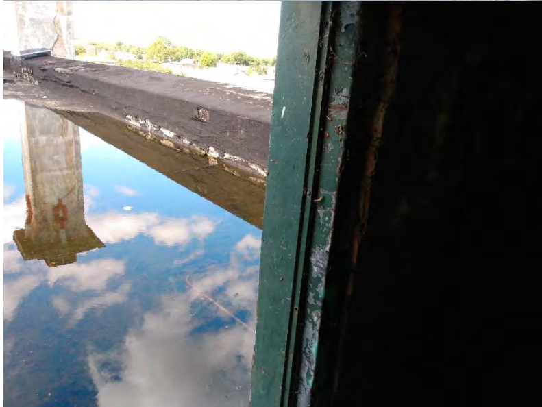
35. Green wooden doorframe to rooftop.
