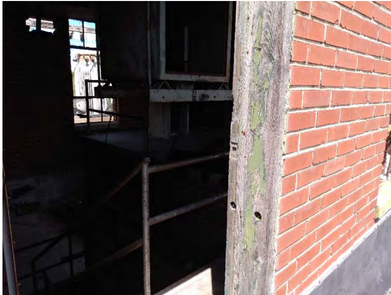
28. Green wooden door frame to rooftop.
