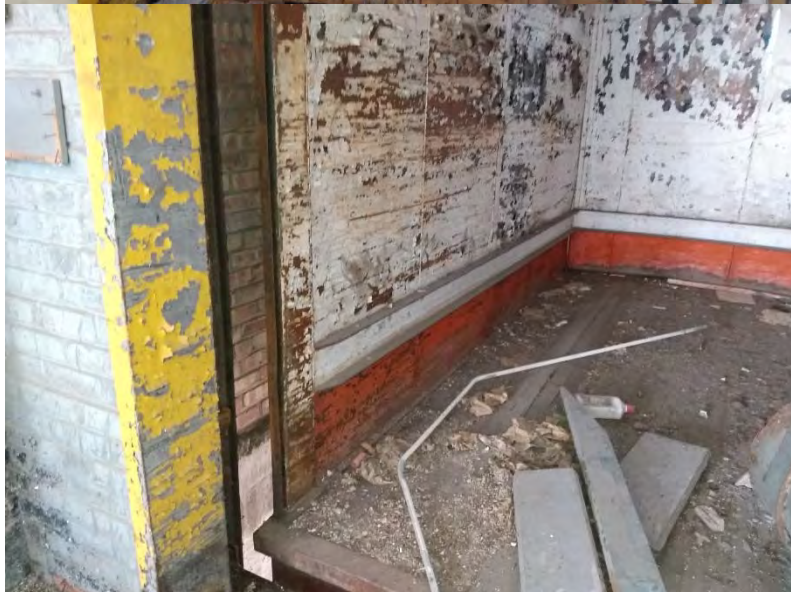
15. Metal, yellow elevator frame and orange metal lower half of elevator cart.
