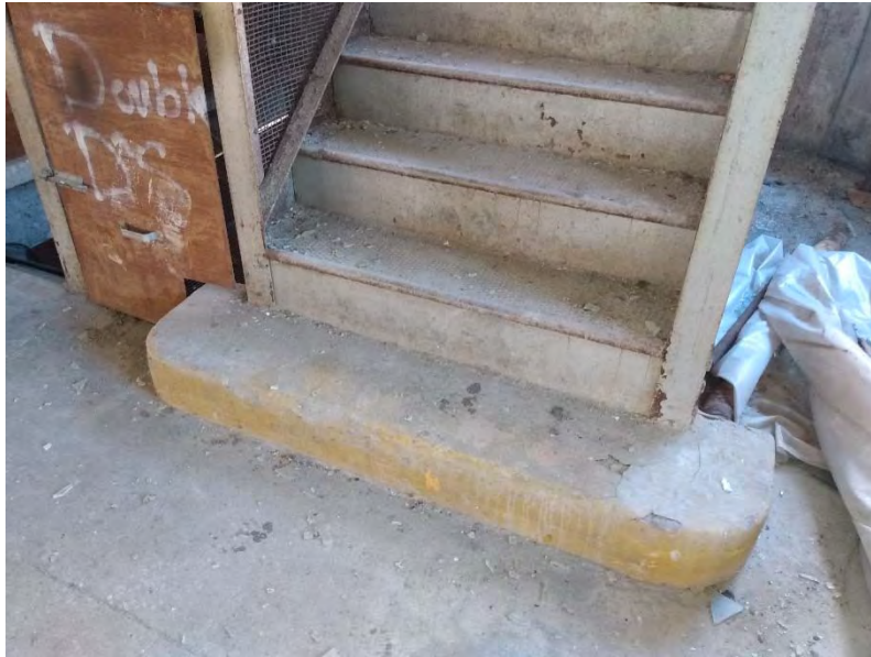
34. Yellow concrete stairwells.
