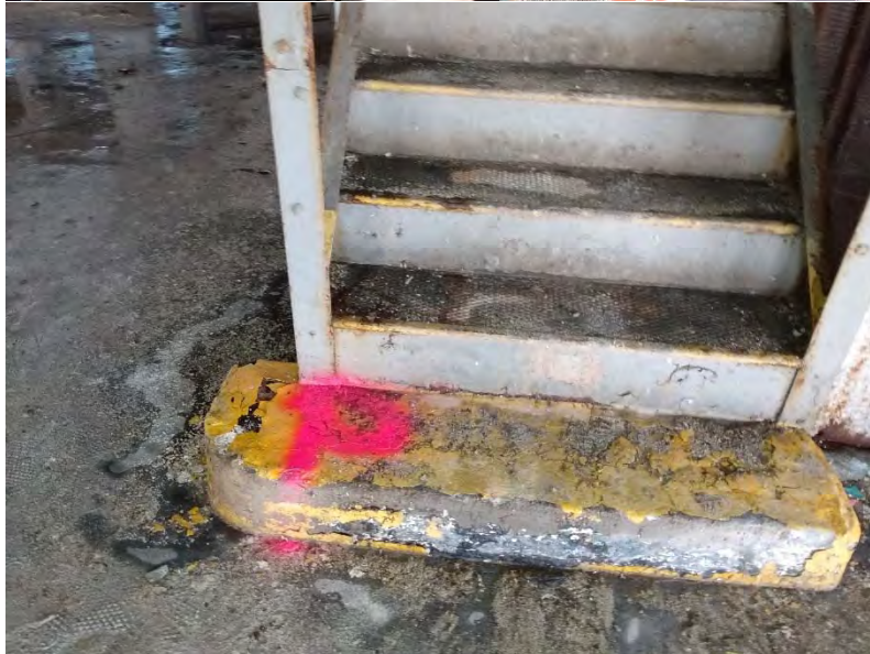
29. Yellow concrete stairwells.
