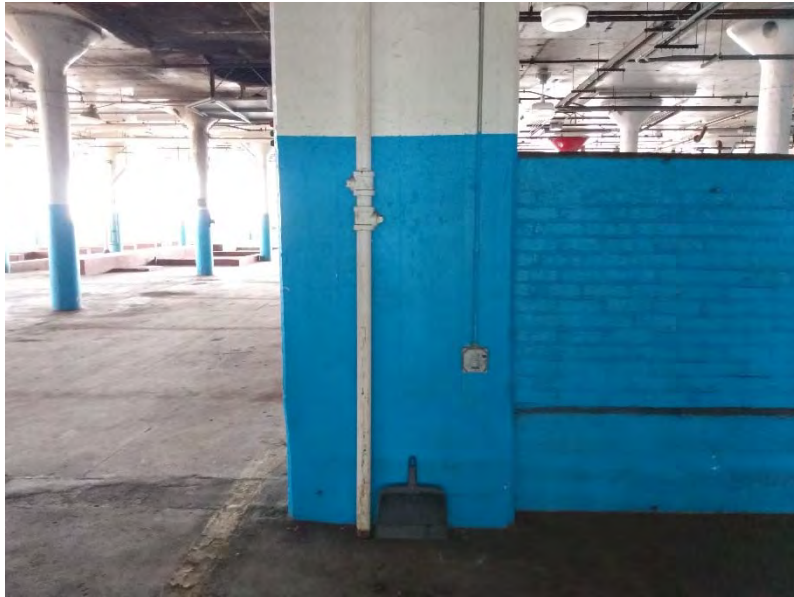
10. Blue on concrete and brick walls.
