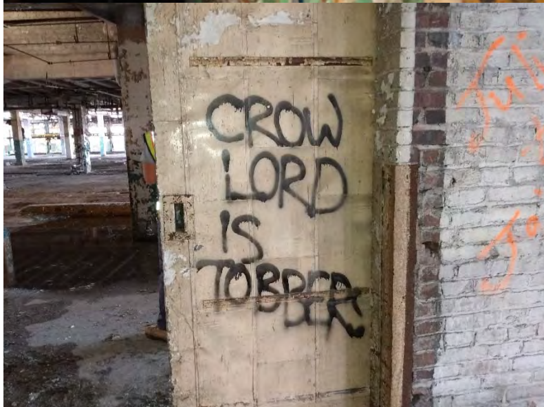
24. Cream, metal fire door.
