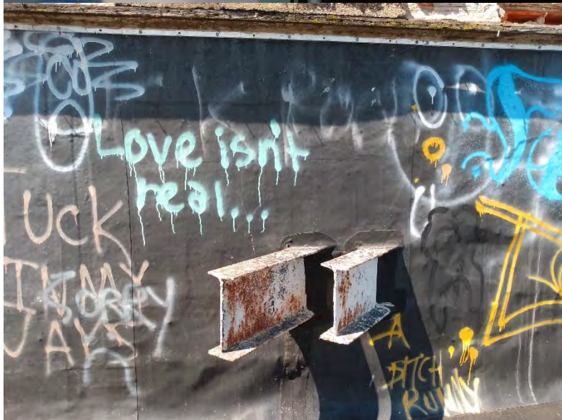
36. White, metal beam on rooftop.
