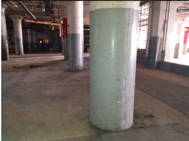
3. Gray lower half of concrete column.
