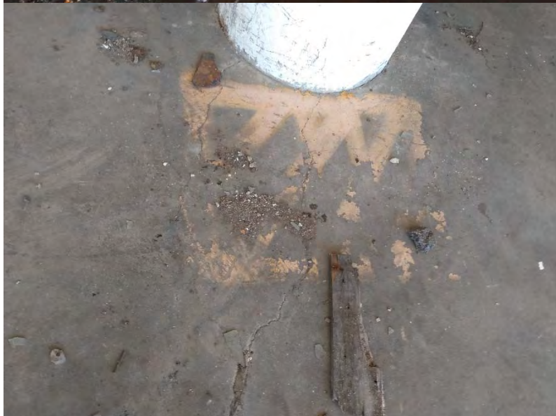
9. Yellow safety zone on concrete floor.
