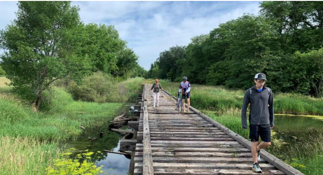
Bridge over an Iowa River oxbow, 6 miles north of proposed trailhead location in Marshalltown
