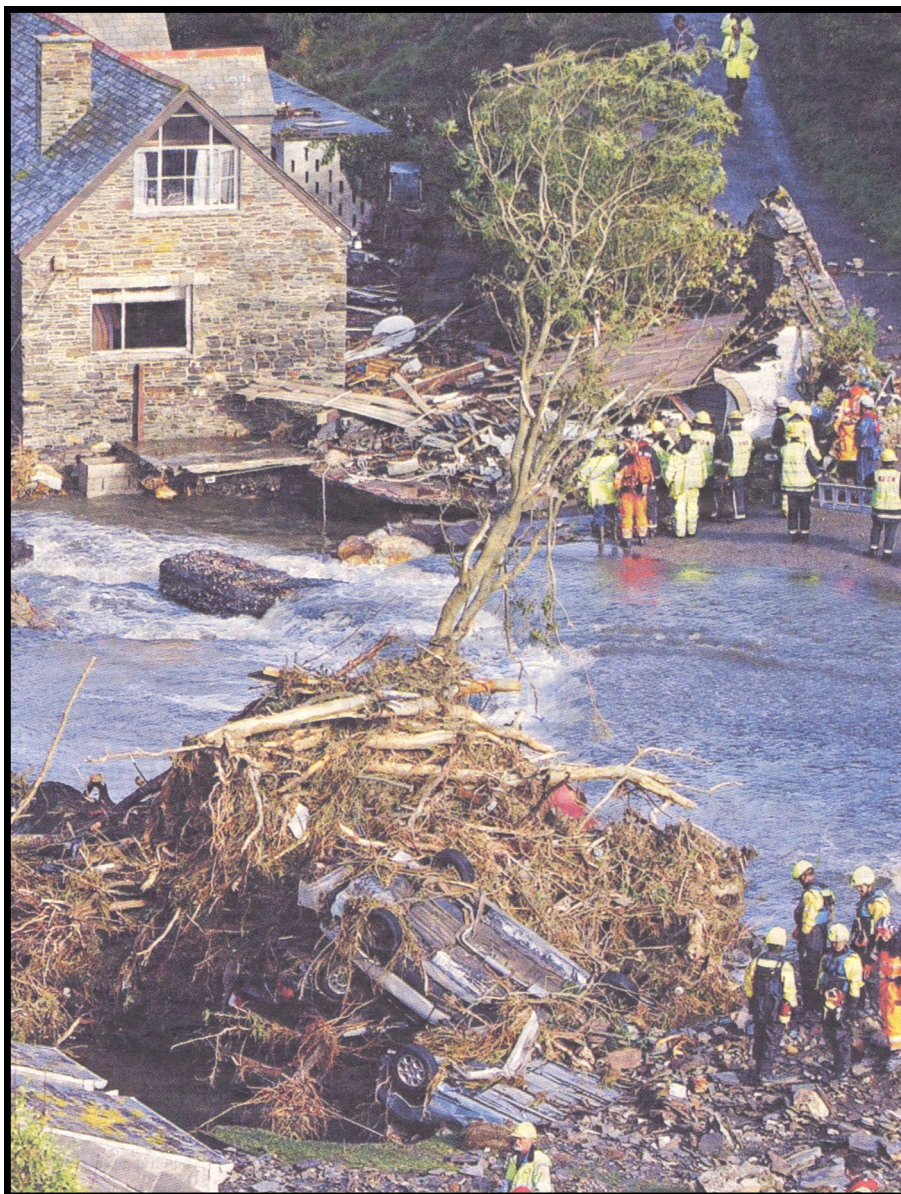
Devastation at Boscastle, Cornwall, after the floods of 16.8.04
