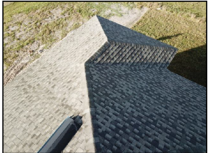
74. Asphalt shingles
