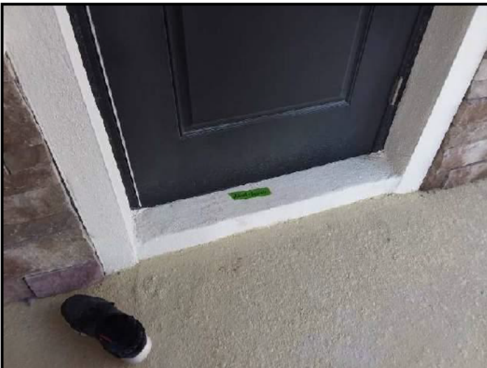
11. Adjustment needed to stucco at threshold
