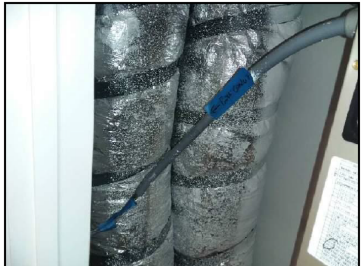
35. Conduit needed - must be complete to wall
