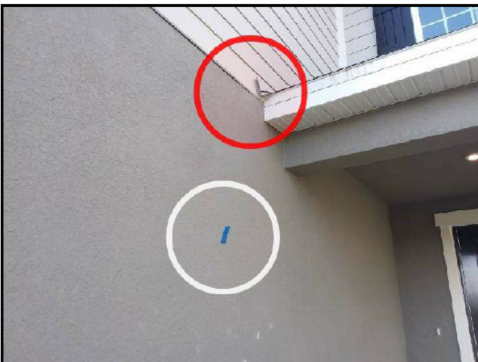
99. Caulking needed behind kickout
