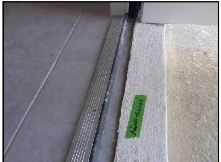
12. Adjustment needed to stucco at threshold
