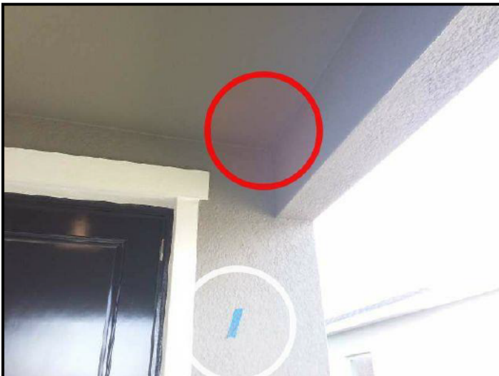
95. Exposed drywall screws
