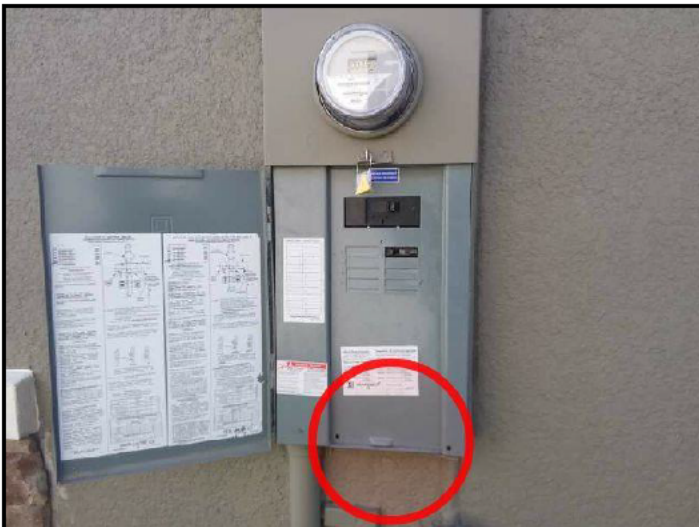
7. Missing fasteners
