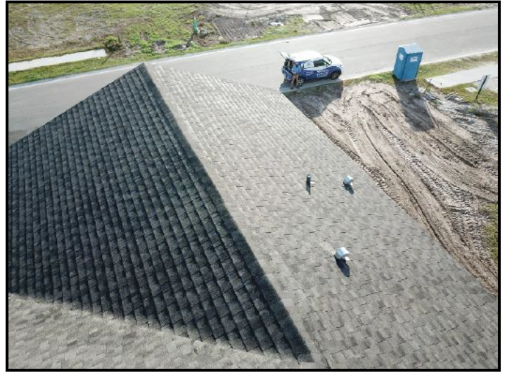
76. Asphalt shingles
