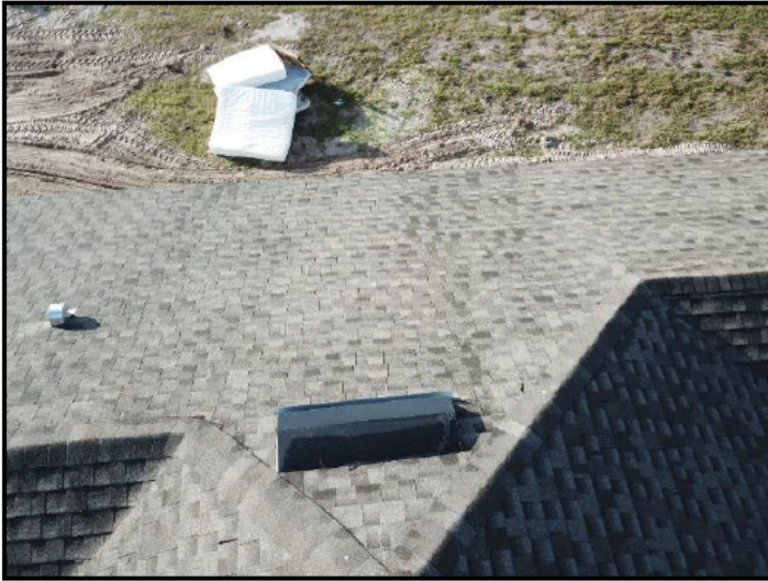
75. Asphalt shingles
