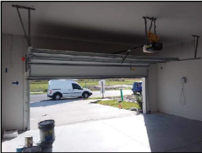
101. Adjustment needed to garage door
