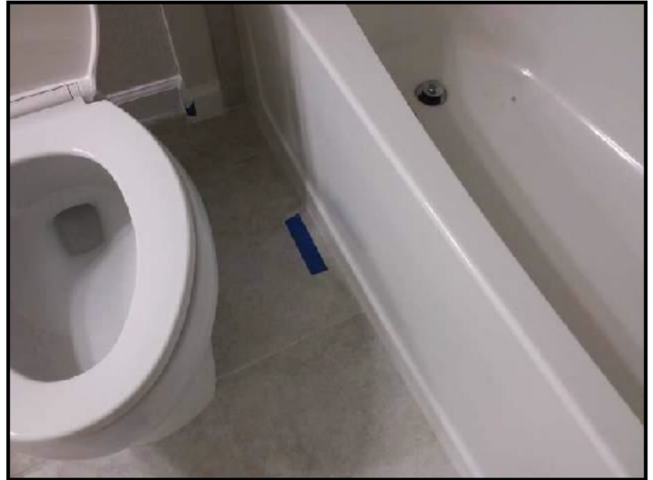
45. Grout cracking
