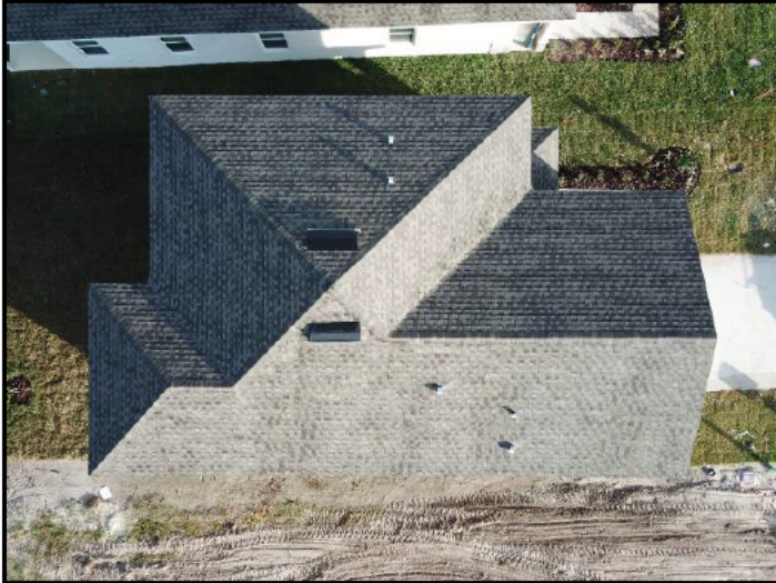
71. Asphalt shingles
