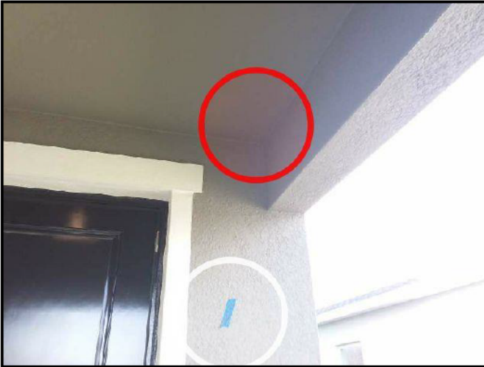
9. Exposed drywall screws
