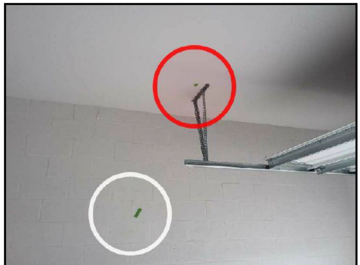
104. Minor damage to drywall
