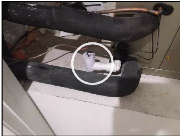
123. Automatic shut-off device in place
