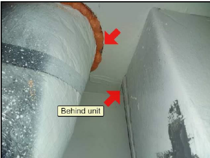
34. Sealant needed around plenum on inside
