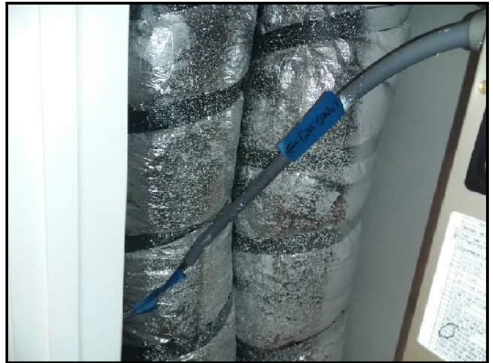
151. Conduit needed - must be complete to wall
