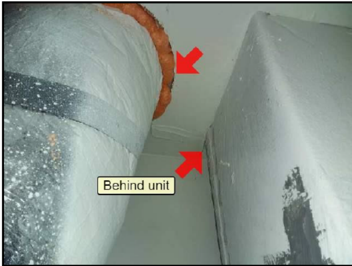
150. Sealant needed around plenum on inside
