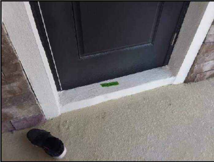
97. Adjustment needed to stucco at threshold
