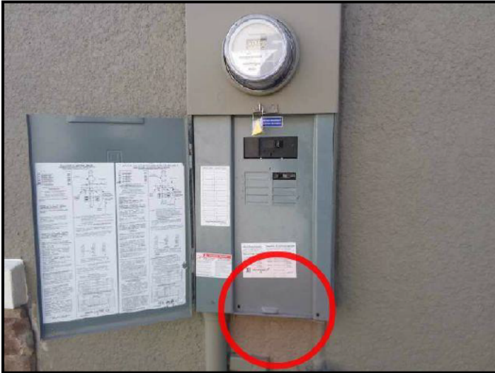
93. Missing fasteners
