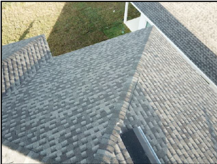
73. Asphalt shingles
