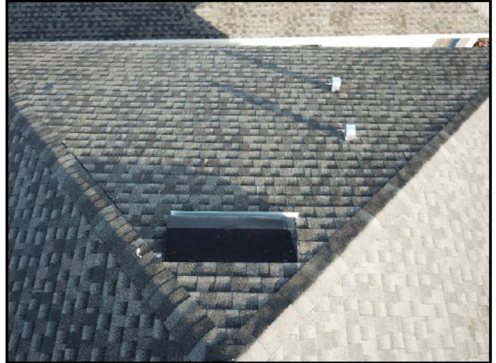
72. Asphalt shingles
