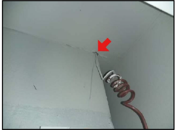
33. Sealant needed around plenum on inside
