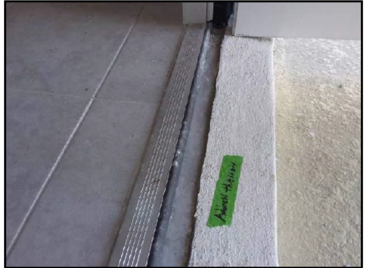
98. Adjustment needed to stucco at threshold
