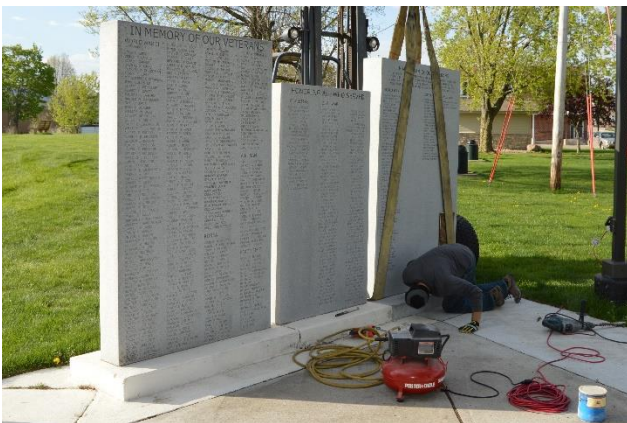
One of the two monuments being set at the park.
