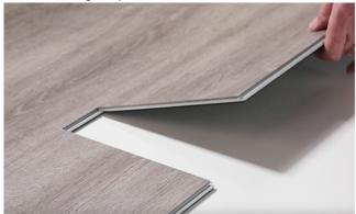
2 Slide the plank until it reaches the short side of the next plank
