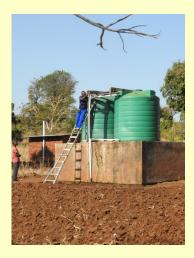
Once again able to return this September, the solar powered downwell pump was installed, two 1,300 gallon tanks were purchased and set in place, and long ditches
