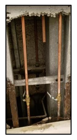
Removing old tiles and opening up the plumbing to install new up to code shower/bath faucet
